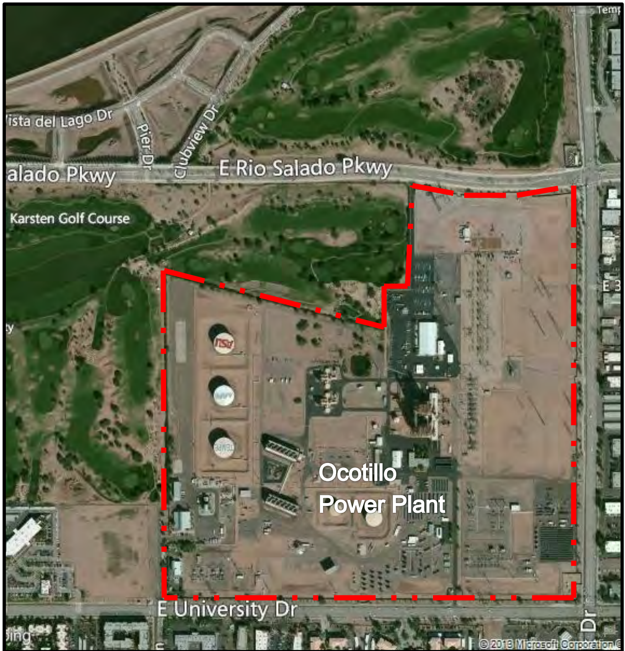
FIGURE 2-2. Aerial image of the existing Ocotillo Power Plant.
